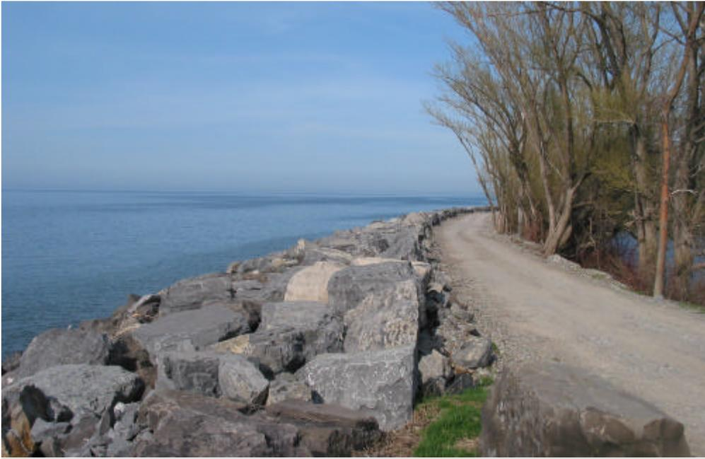
1. Successfully closed out the Port Bay Improvement Program Economic Development Initiative Grant (pictured above) in the amount of \$319,125. Project resulted in the construction of 1,490 linear feet of revetment successfully controlling erosion on the barrier bar and opening it to recreational activities after a long absence. (Sharon Lilla)
