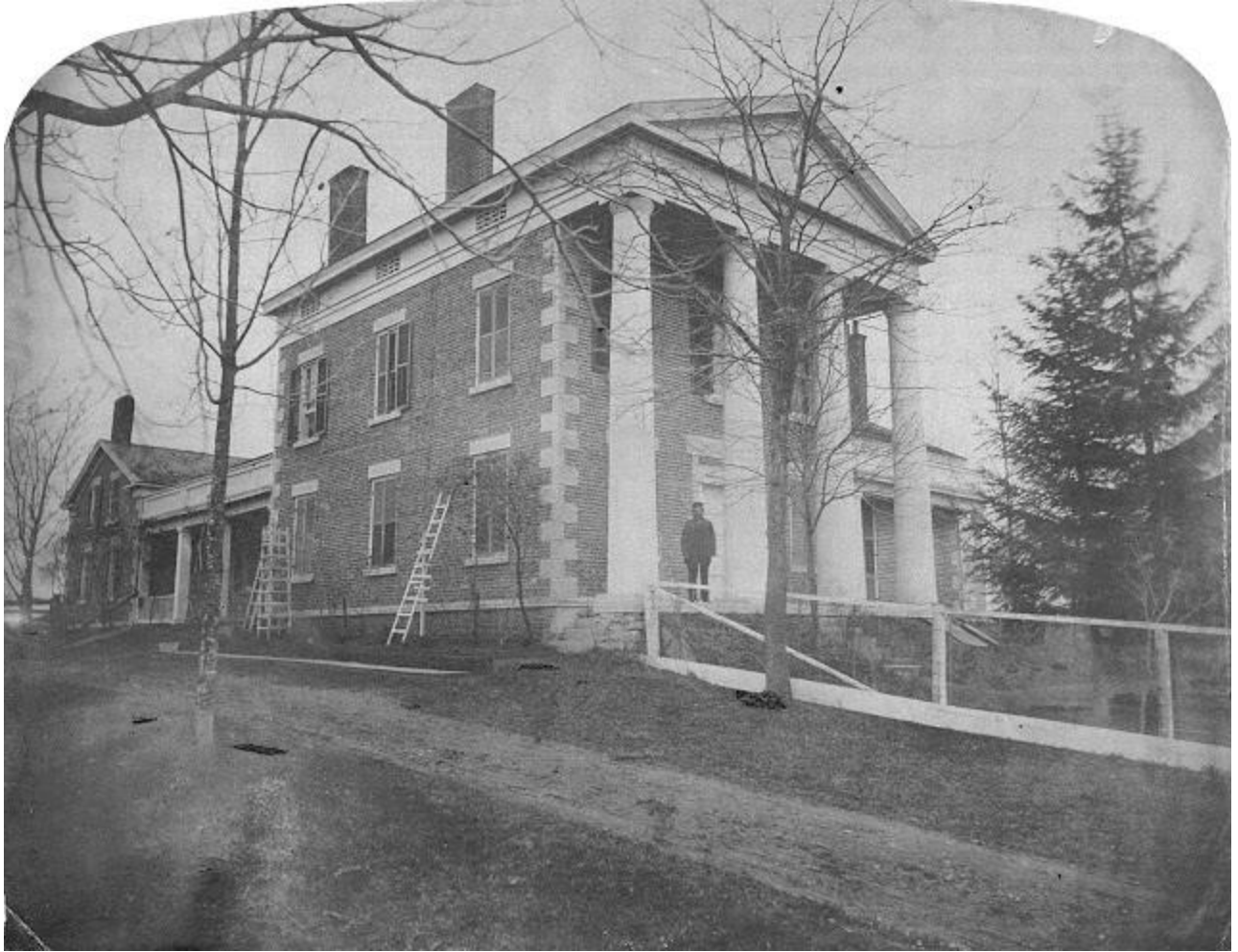
The stately James P. Bartle cobblestone farmhouse was built on what is now West Miller Street in Newark in 1836. Bartle operated the first store in Newark He was a veteran of the War of 1812 and was a prominent businessman. The house was demolished in 1938 to make way for the new junior high school. Photo, taken in the 1870s, courtesy of Newark-Arcadia Historical Society.
